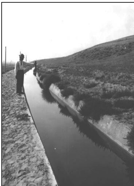
Irrigation flume, Kamloops (BCA F-08001)
